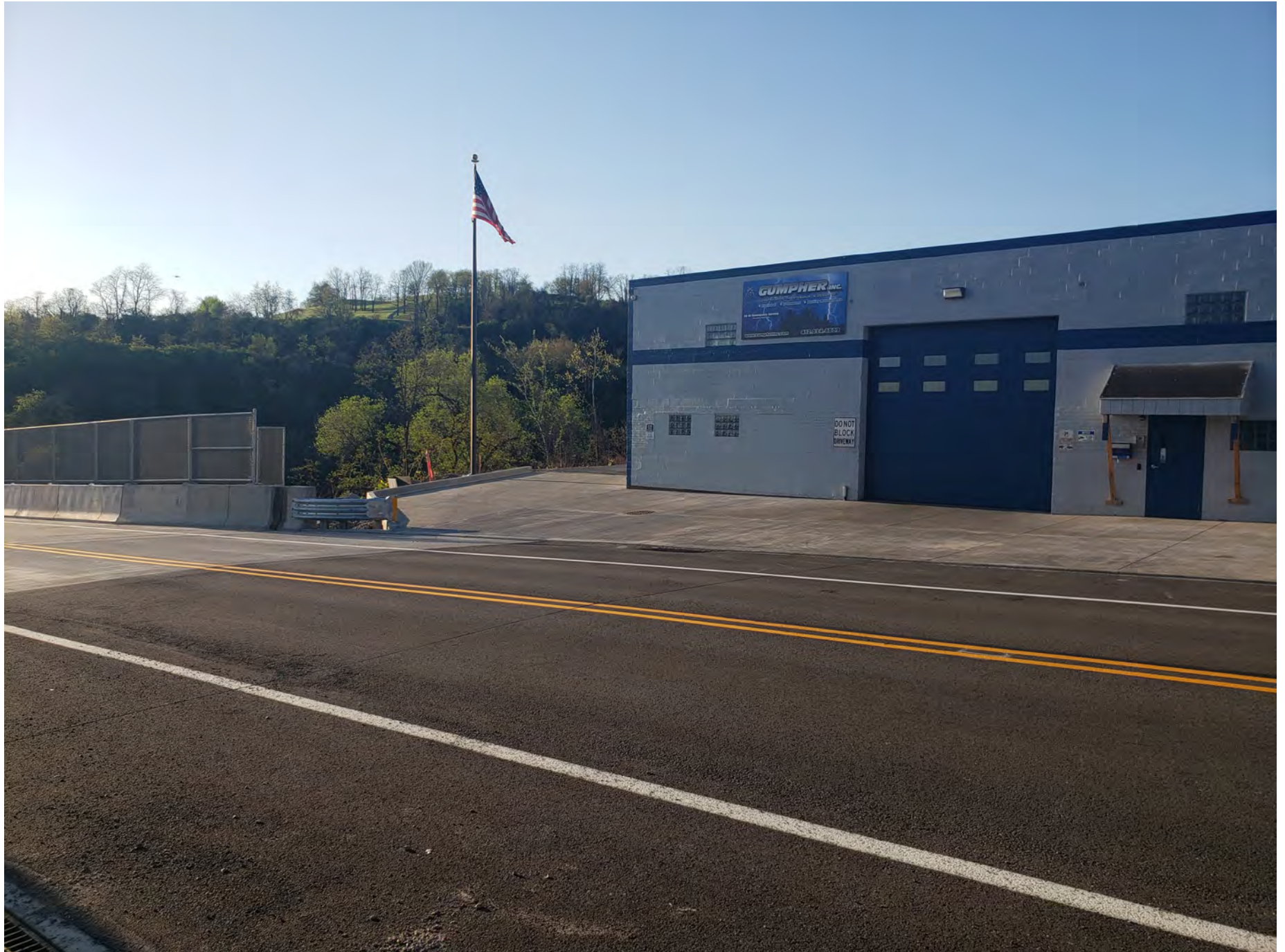
05 - Proximity of Adjacent Local Business to New Bridge
