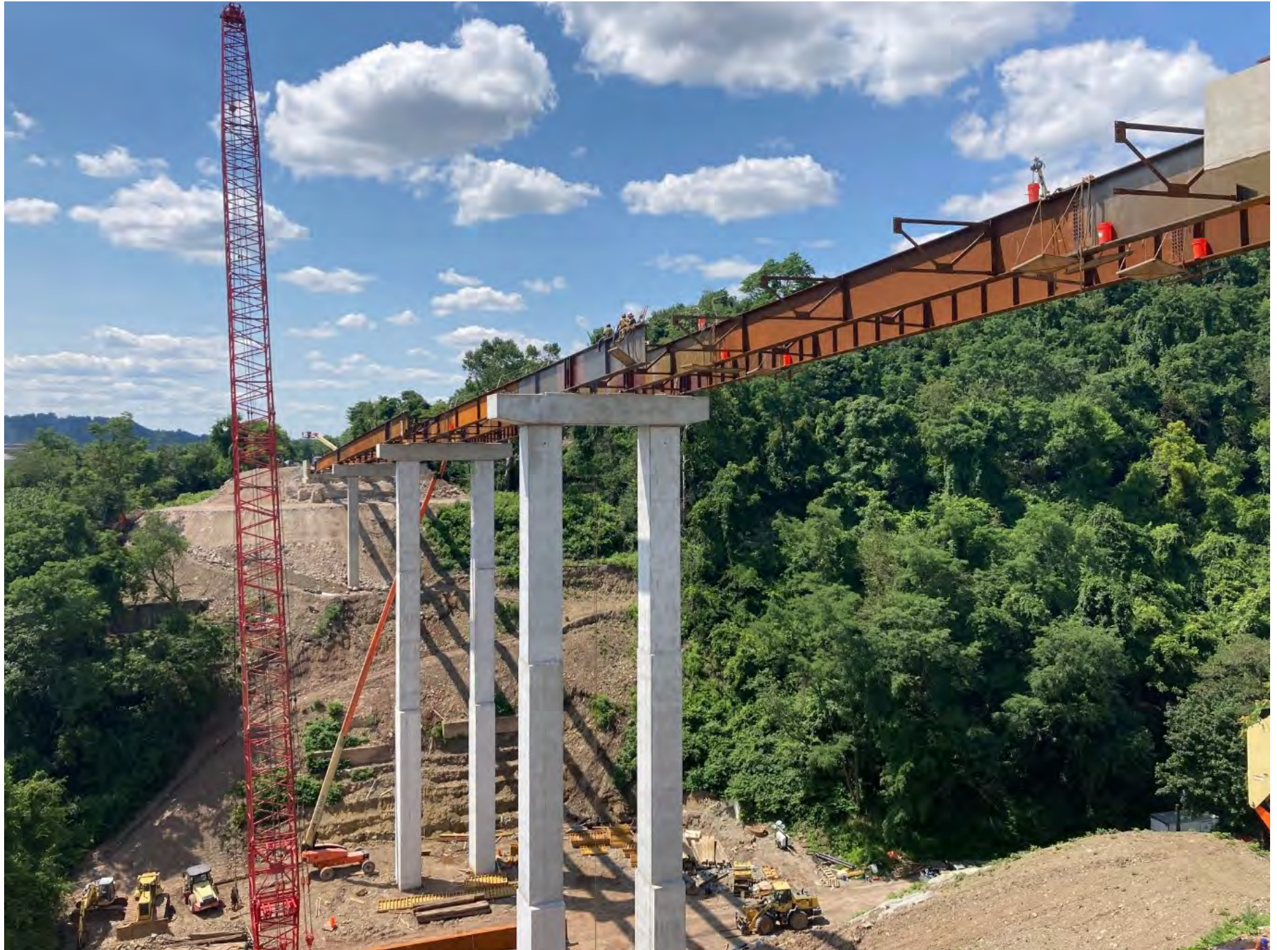
04 - Girder Erection over the Valley
