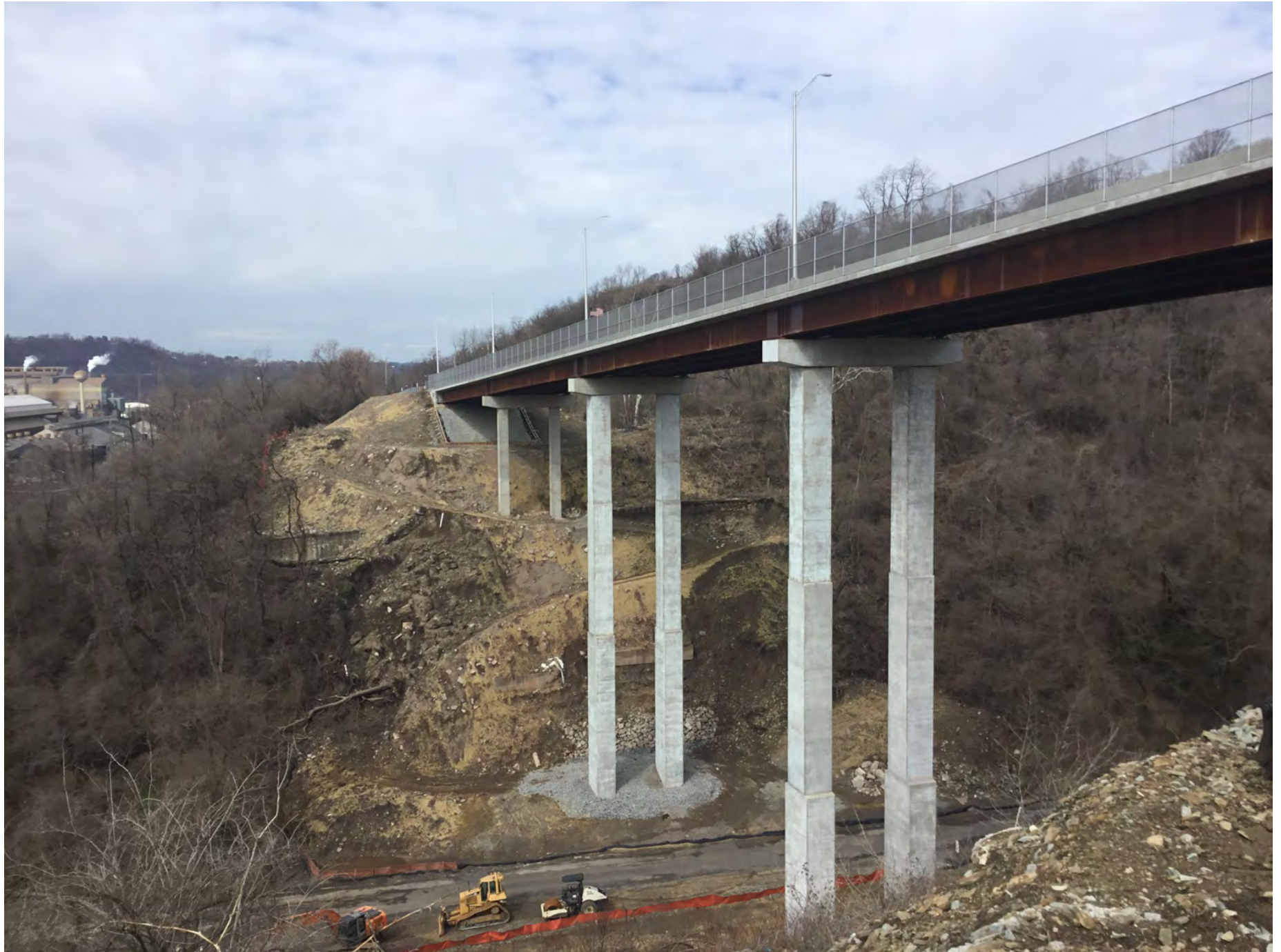
01 - Completed Dooker's Hollow Bridge
