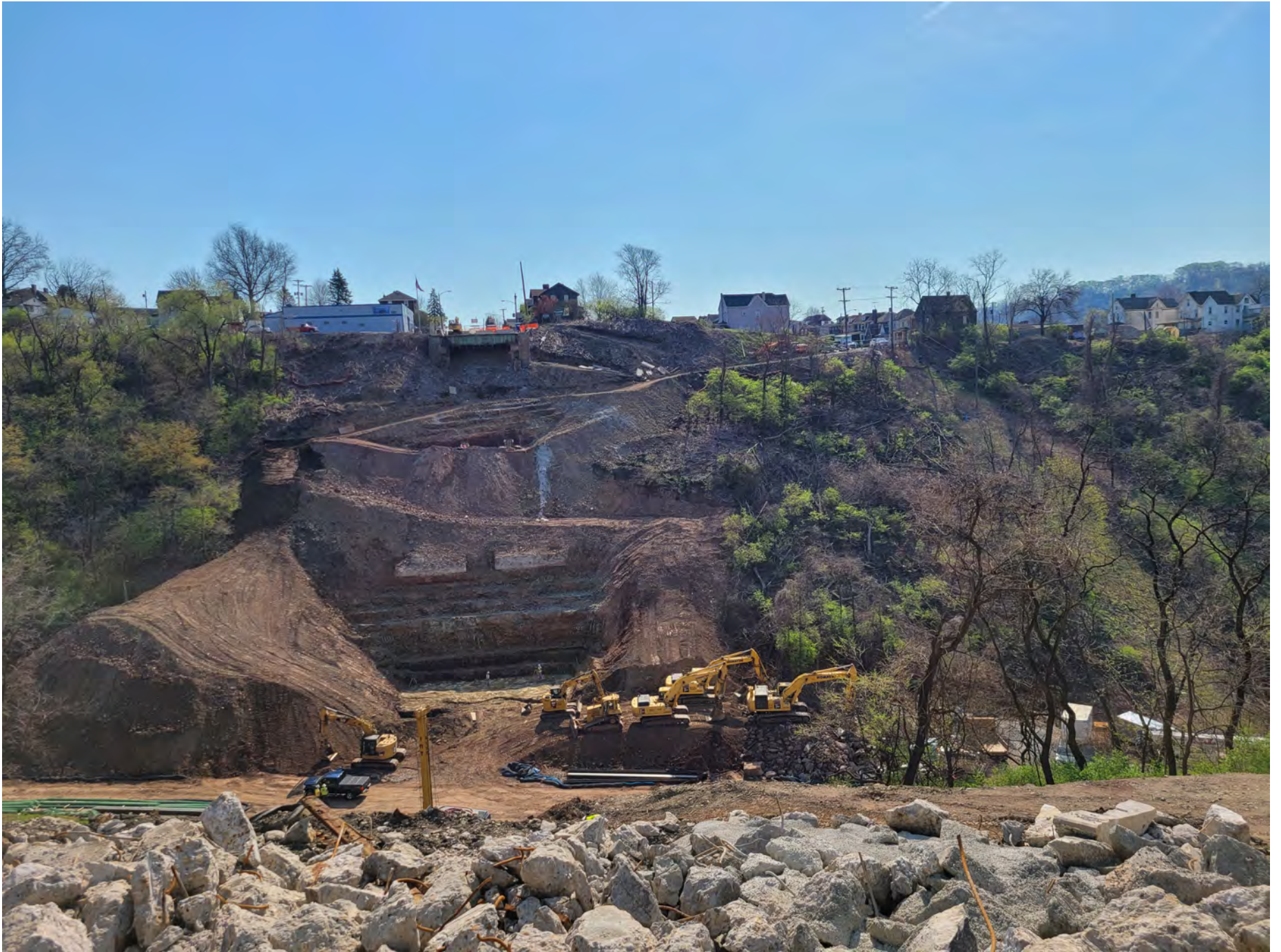
03 - Earthmoving Required on Steep Hillside
